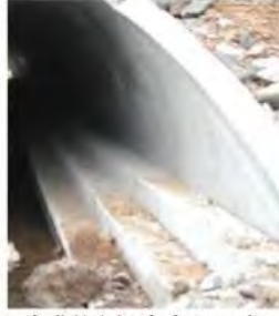
Illustrations of suitable ledges for fauna crossing
